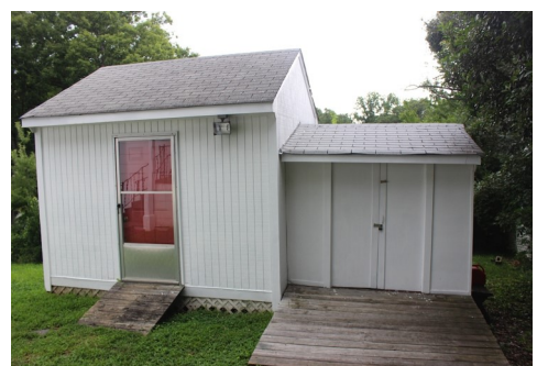
Workshop & storage sheds..
