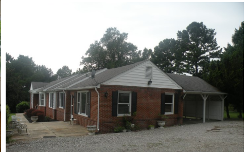
Carport on rear of home.
